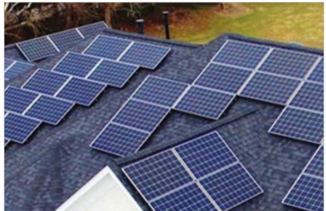
Traditional Solar Panels
