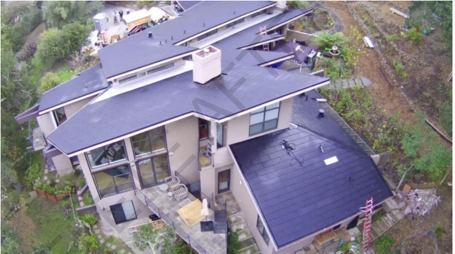
Finished installation for reference:
