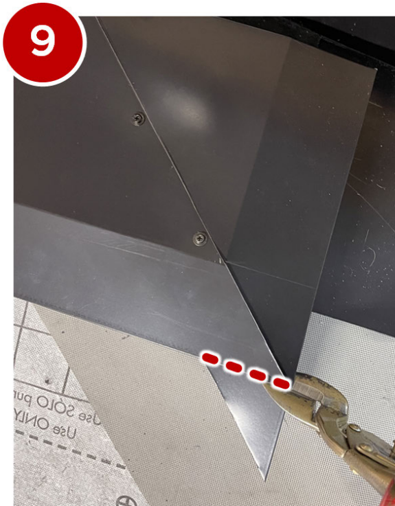
Final view of tab / transition flashing:
