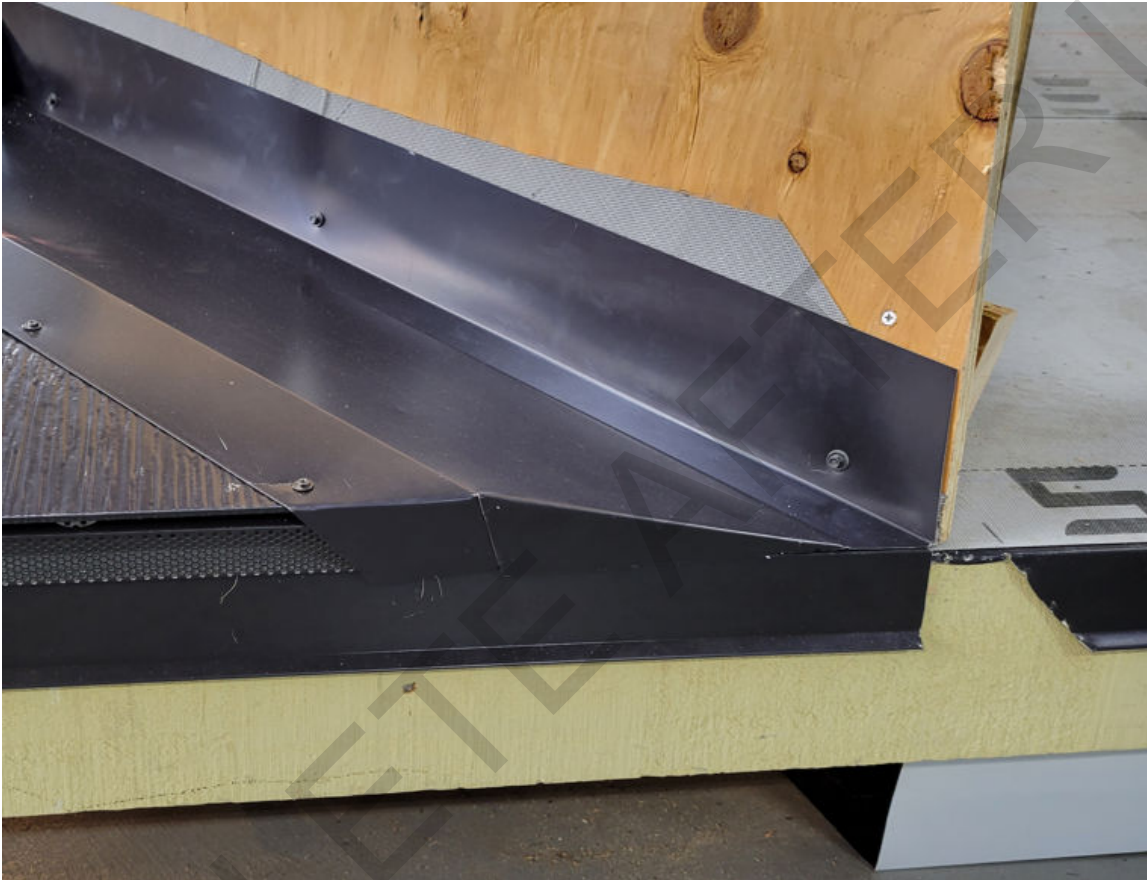
Finished installation for reference
