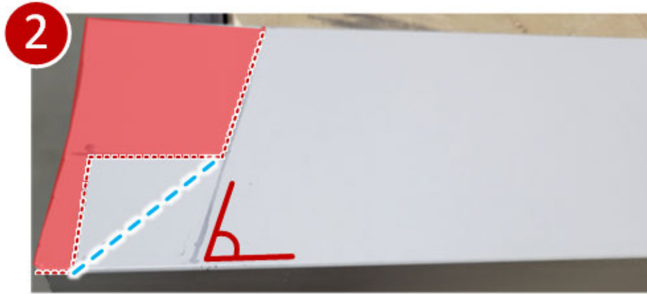
Image showing the back of the wall flashing
