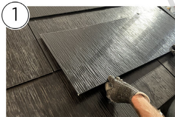
Pictured: tile skin (1a) placed over a metal tile (1b) .
