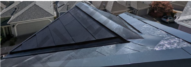
Finished cut and tuck method installation for reference:
